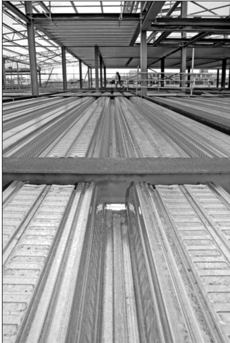
**Figure 7.5** View of Slimflor construction using ComFlor 225 decking.
