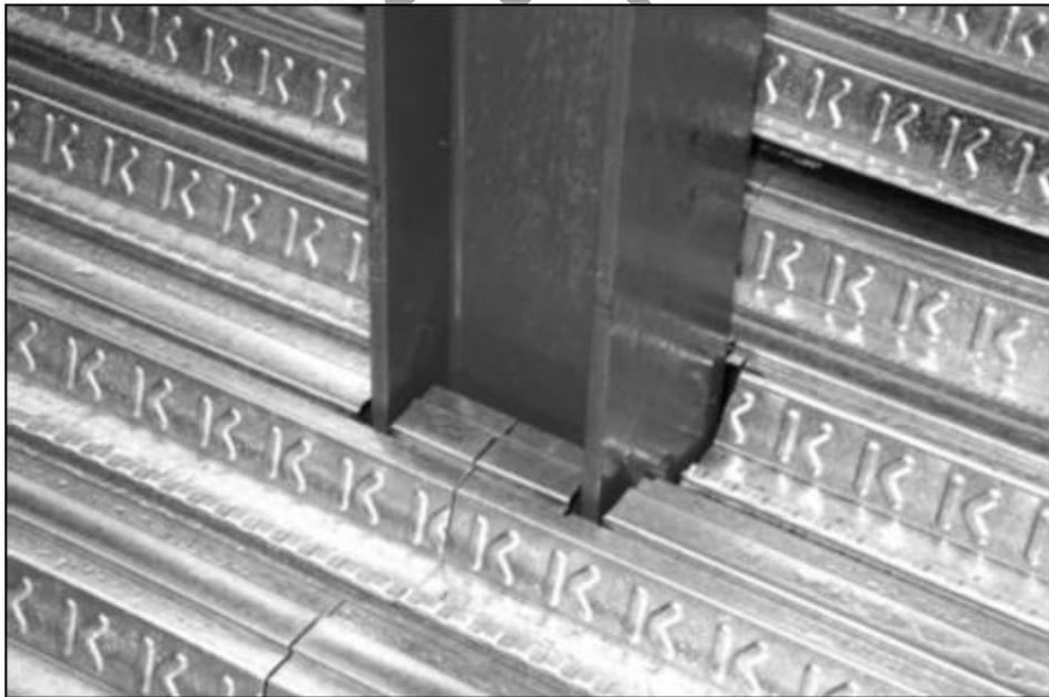
**Figure 4.9** Typical detail of decking installation around a column
