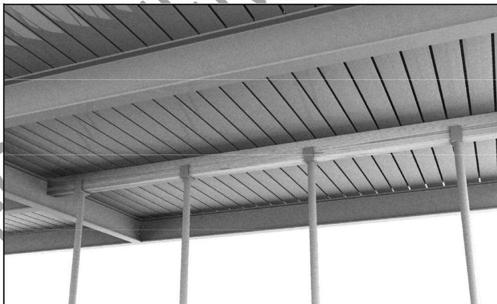
**Figure 4.17** Temporary support using an 'Acrow' props
