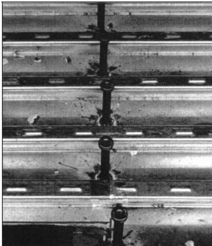
**Figure 5.7** A typical run of stud shear connectors
