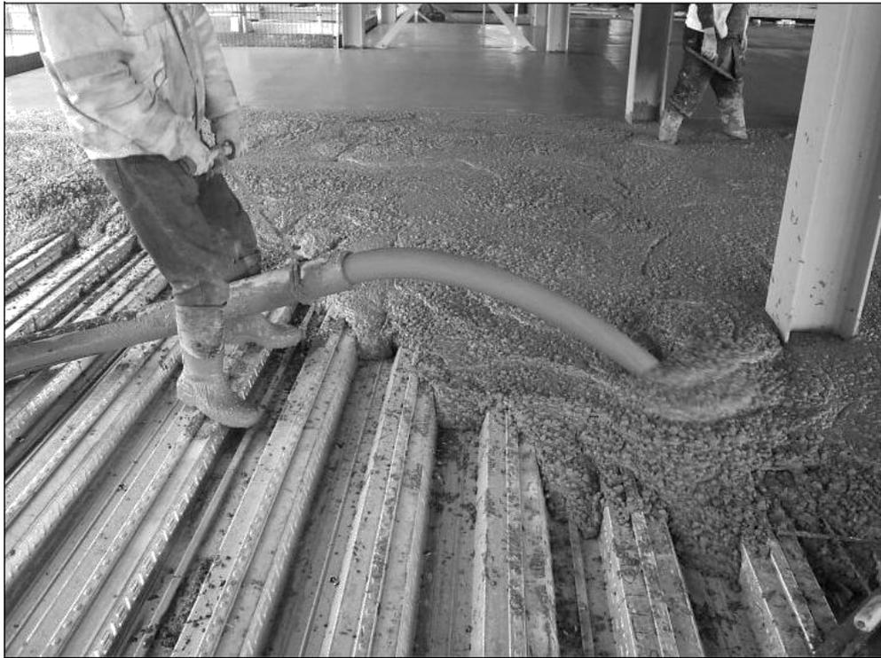
**Figure 6.4** Pumping of fibre-reinforced concrete
