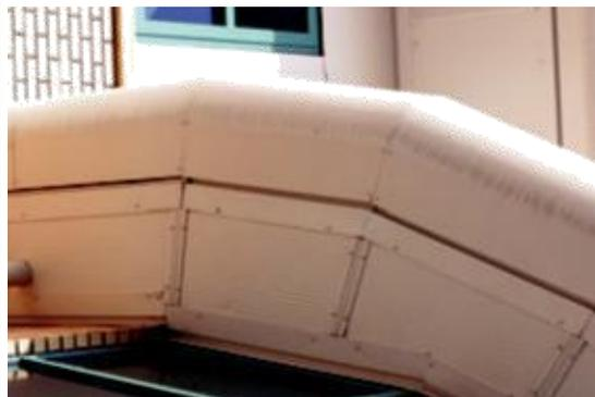
Where two bull nose fabrications meet, a pre-fabricated bull nose corner provides a neat pre-engineered detail.
