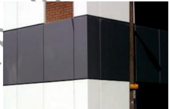
These are manufactured from the same panels that make up the wall cladding system of the building. They enable a continuous clean line around a corner which has the effect of making the cladding look as if it is a continuous piece rather than joined together.
