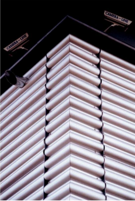
These corners are made to suit both built-up systems and composite panel cladding systems.
