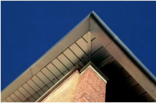
Fascias are used on vertical faces and soffits for the underside of horizontal faces. These items can be considered as either cladding and fabrications, however they are mentioned here because they are often used to create architectural features to complement or contrast with the main cladding system used.
