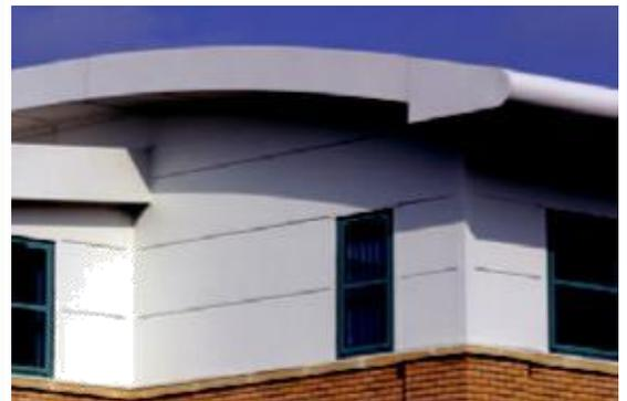
These are used, for example, to provide the end detail to a curved roof. The range of applications is extremely wide, however the curved fabrication almost inevitably makes a strong aesthetic statement.
