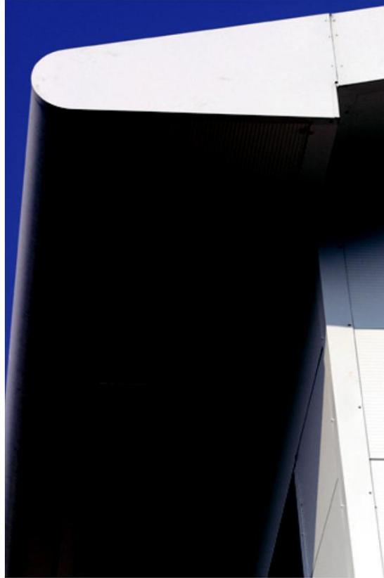
Circular curved fabrications used to create a rounded feature on a building; they are often used on the eaves.
