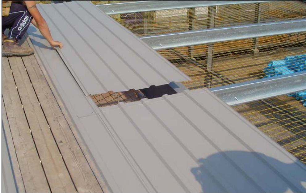
**Figure 5.5** *Liner sheet installation progressing into the span of the purlins with the installer working from a 'Youngman' board*
