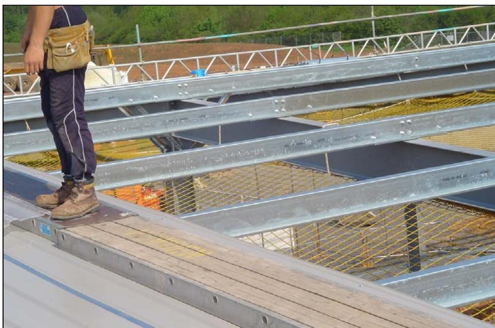
**Figure 5.3** *Safety nets and guardrail in place during roof cladding installation* (Image courtesy of C A Roofing)
