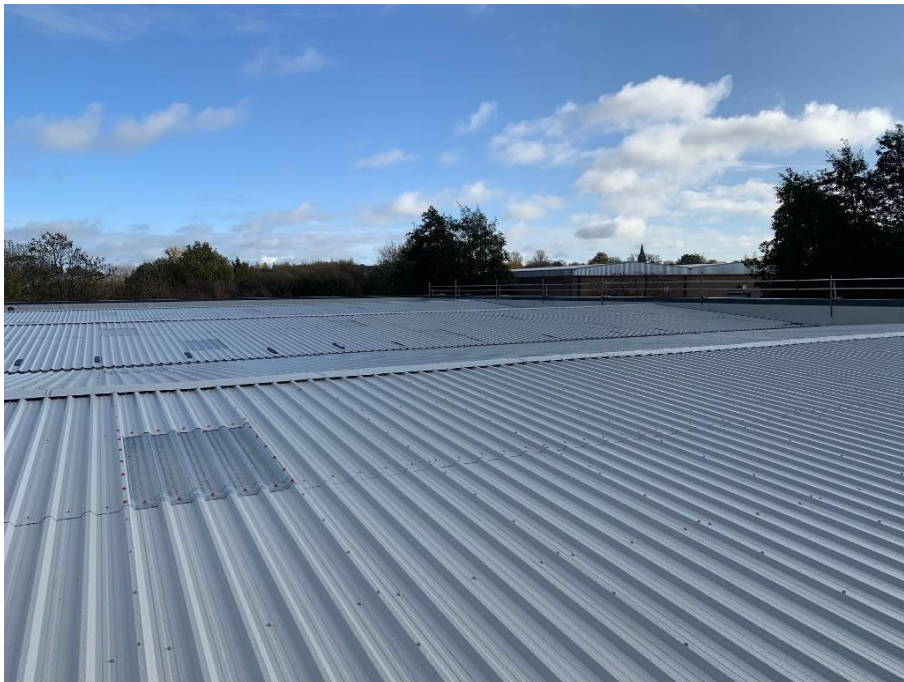
Fig 3: Completed over roof using a profiled metal outer sheet and integrated rooflights
