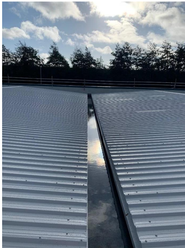
Fig 6: Completed profiled metal over roof incorporating membrane lined gutter system
