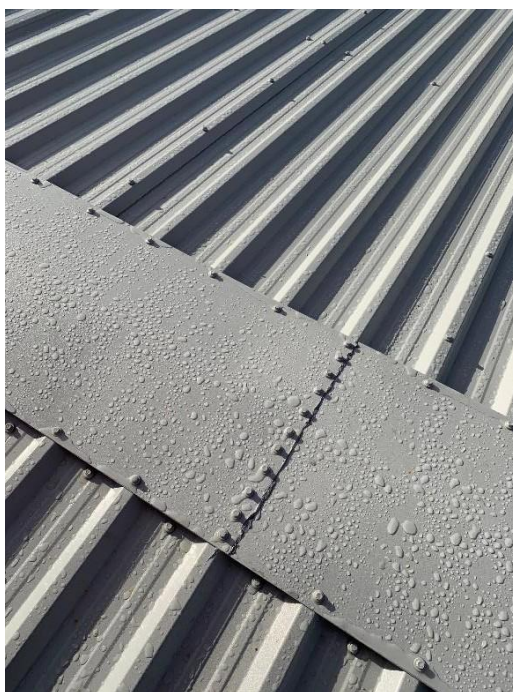
Fig 5: Fully integrated sealed flashing incorporating flute fillers
