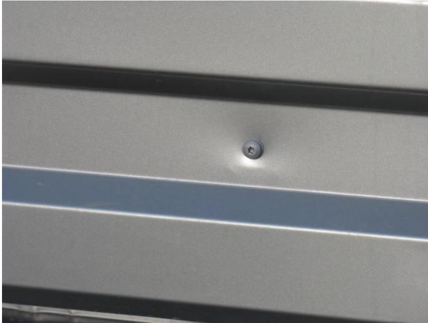
Fig 8 Example of an over tightened fastener
