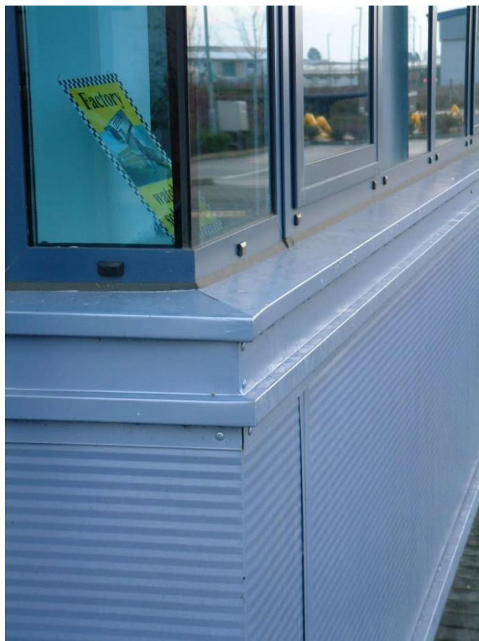
Fig 3 Showing consistent colour match between the panel and the flashing
