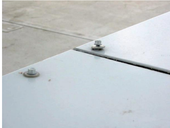
Figure 8: Consequence of no movement allowance at fastener location: fastener backing out of a capping
