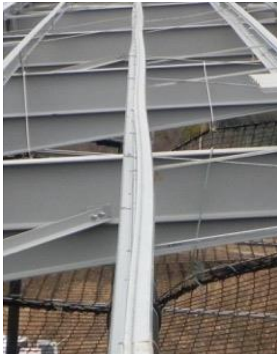
Excessive purlin rotation before any load applied
