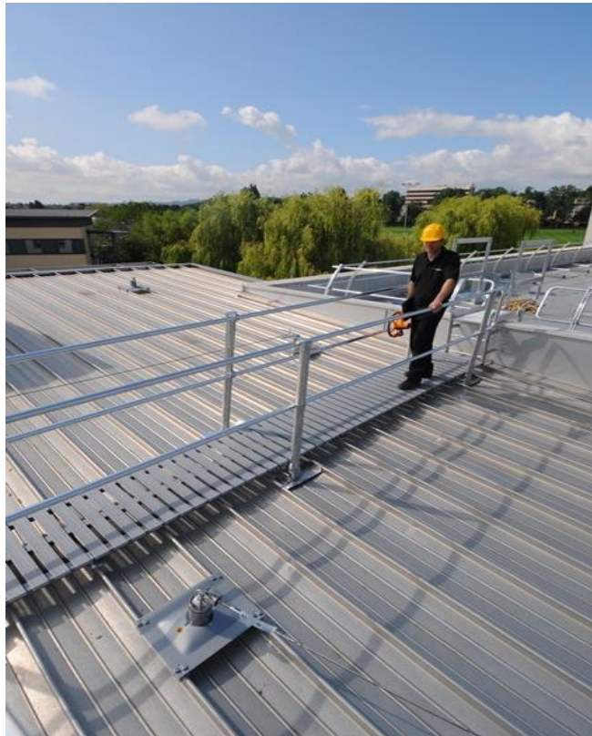
Collective fall protection of guardrail and walkway with accompanying cable system providing access to restricted areas
