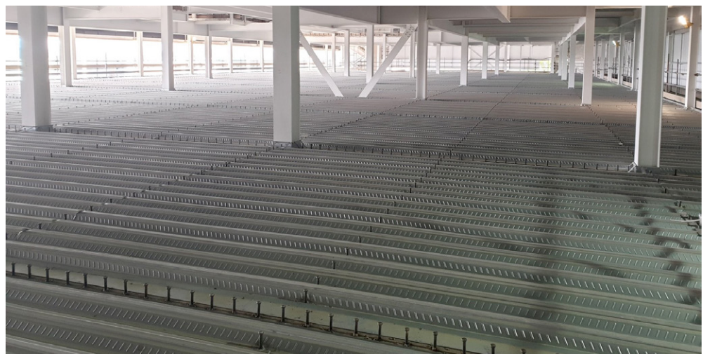
Figure 1.1 A typical example of composite floor construction, showing decking placed on a steel frame
