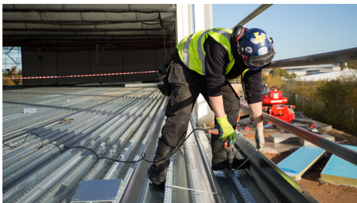
Figure 4.16 Setting out of edge trim
