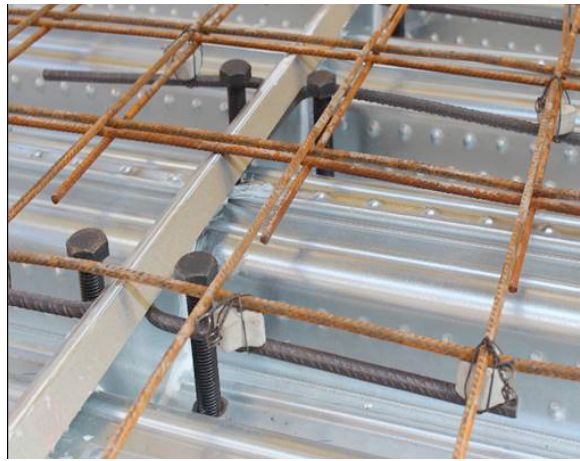
Figure 7.2 Partial depth edge trims and U-bar details
