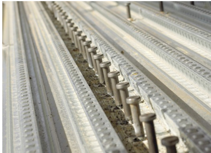
Figure 5.8 A run of stud shear connectors
