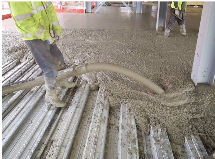
Figure 6.4 Pumping of fibre-reinforced concrete
