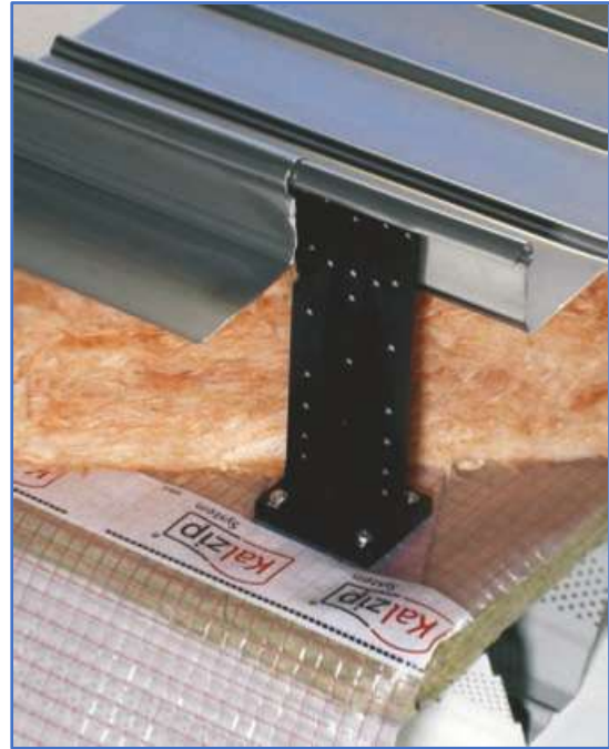
Figure 8.8 – Mesh reinforced vapour control layer in a built-up acoustic roof system with perforated decking)
