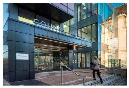
Architectural Profiles' Slimwall CPS aluminium rainscreen system was specified for the redevelopment of Trowbridge County Hall to provide a retrofit building envelope which could achieve a 40 per cent reduction in carbon emissions. The building has achieved a BREEAM 'Excellent' rating.
