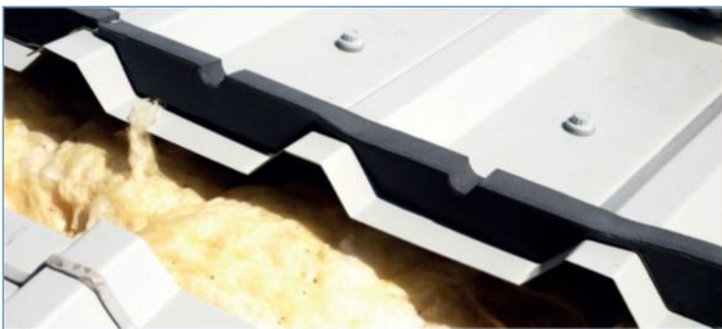
Figure 8.6 – 'Ventilated' profiled ridge filler prior to installation of ridge flashing)
