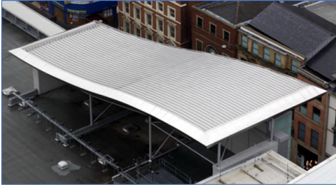
Figure 6.1 shows a standing seam roof system produced from stainless steel coil
