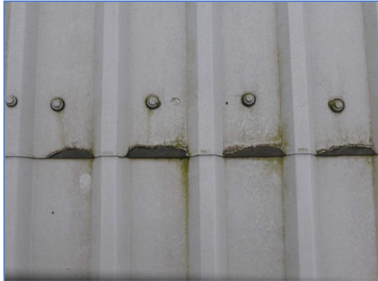
Figure 5.3 – Cut edge corrosion and premature breakdown of paint system at roof end lap detail
