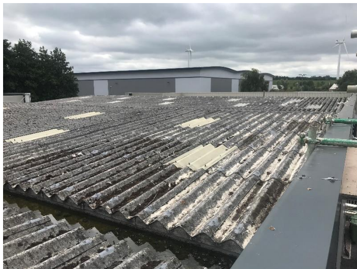
Fig 4: Single skin fragile roof covering with single skin integrated rooflights
