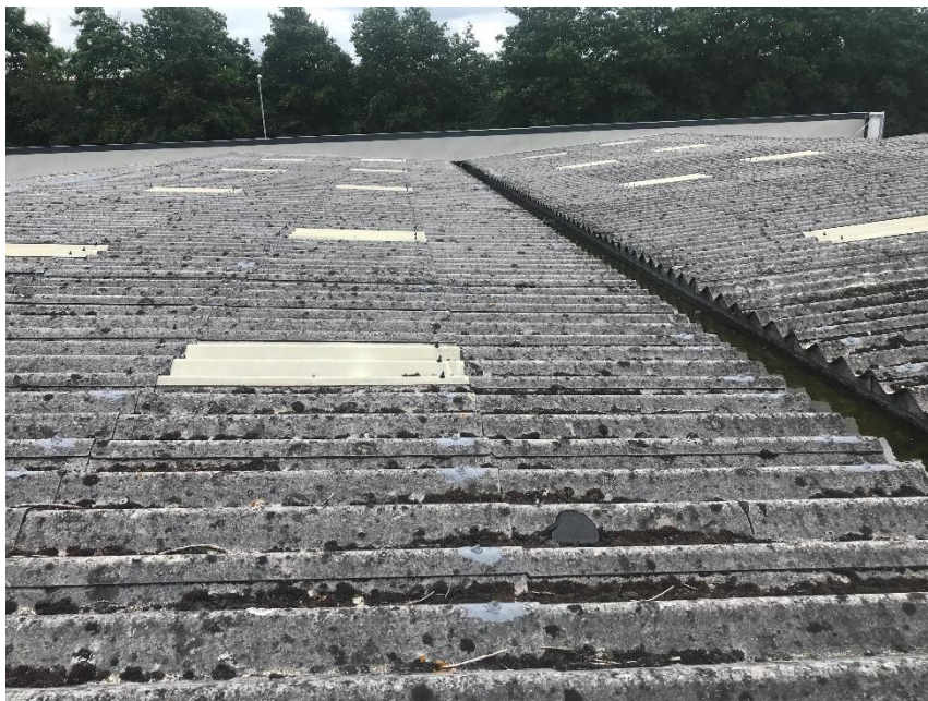
Fig 1: Single skin fragile roof covering before over roofing
