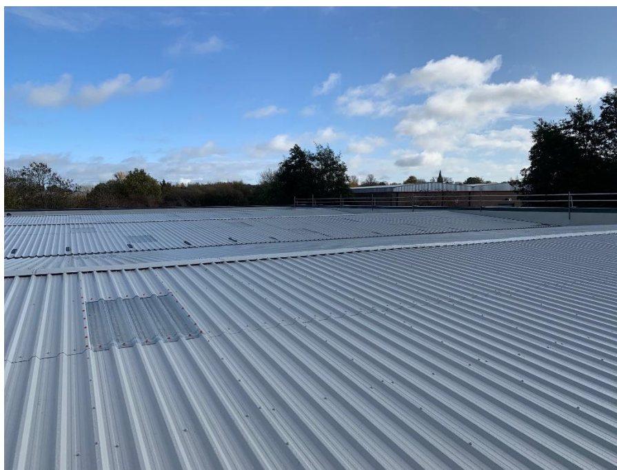
Fig 3: Completed over roof using a profiled metal outer sheet and integrated rooflights
