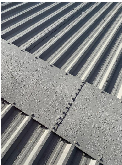
Fig 5: Fully integrated sealed flashing incorporating flute fillers
