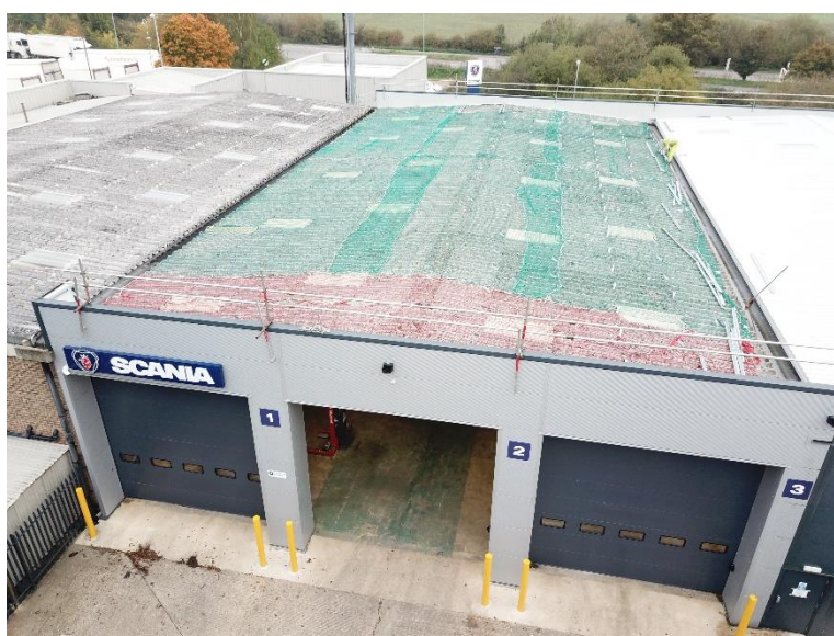
Fig 2: Low pitched single skin fragile roof at the early stages of refurbishment prior to the installation of a profiled metal outer sheet and insulation to comply with current Building Regulations
