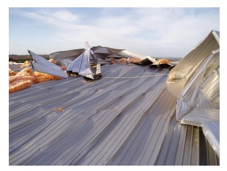
Wind damage: Proper attention to design and detailing will avoid an outcome like this!
