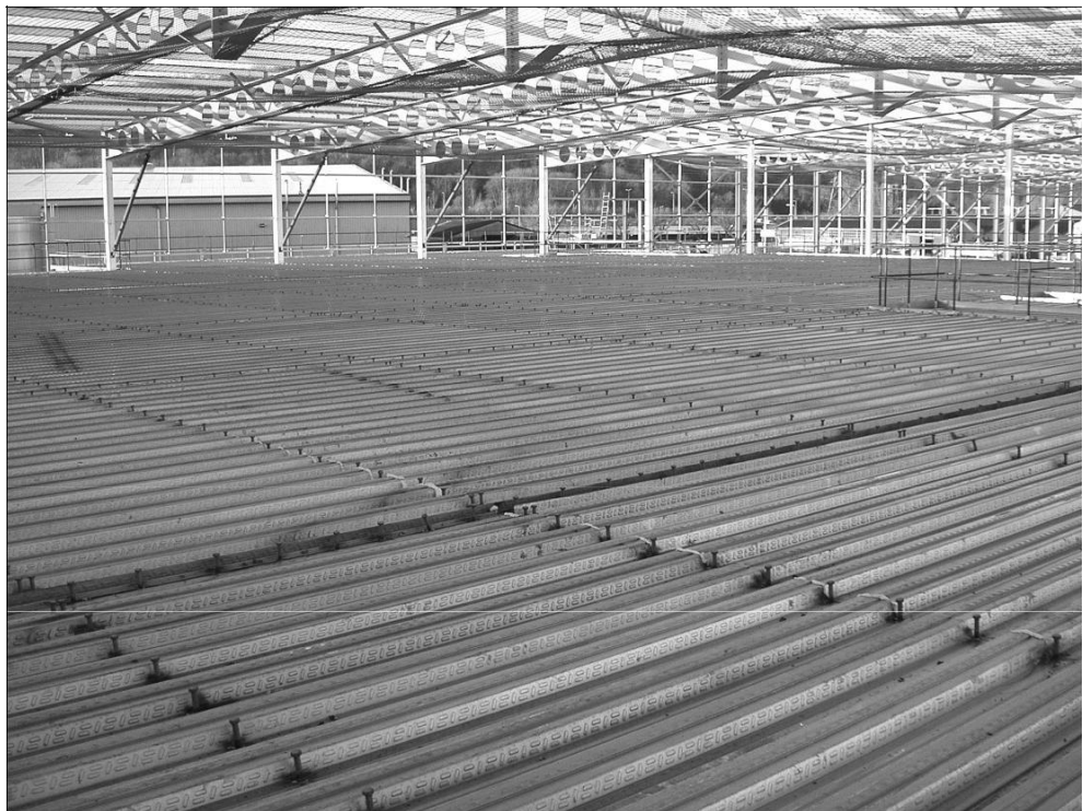
Figure 1.1 A typical example of composite floor construction, showing decking placed on a steel frame
