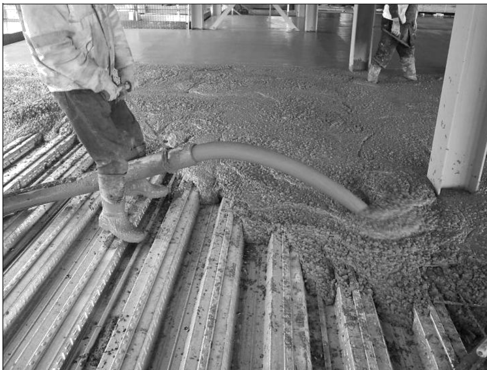
Figure 6.4 Pumping of fibre-reinforced concrete
