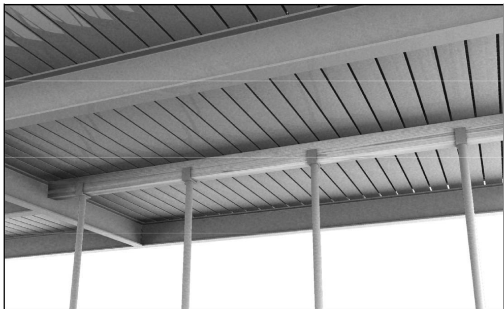
Figure 4.17 Temporary support using an 'Acrow' props
