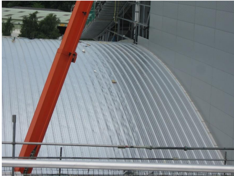
Fig 5 An example of oil canning due to radius of standing seam aluminium.
