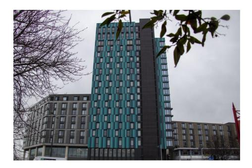
Some 5,500 square metres of Optima TFC in solid aluminium PPC has been used in the construction of Sheffield's New Era Square residential building in Sheffield.
