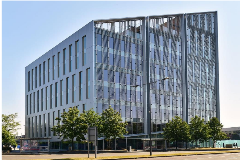
Sotech Optima's secret fix rainscreen cladding system used on Brunel Place, Slough
