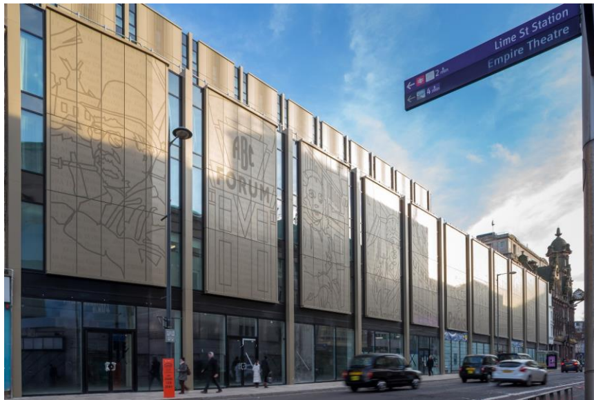
Ash & Lacy's perforated metal façade system -the Gateway Scheme, Lime Street, Liverpool
