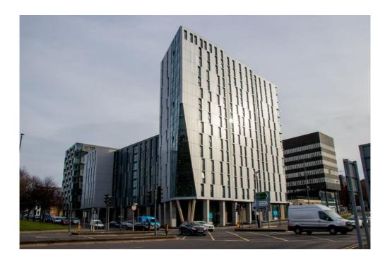
Some 6,500 square meters of Optima TFC in 2.0mm Reynolux Pre-Coat and 2.00mm aluminium Axalta PPC has been used in the completion of the £36 million student accommodation on Norton Street, Liverpool.
