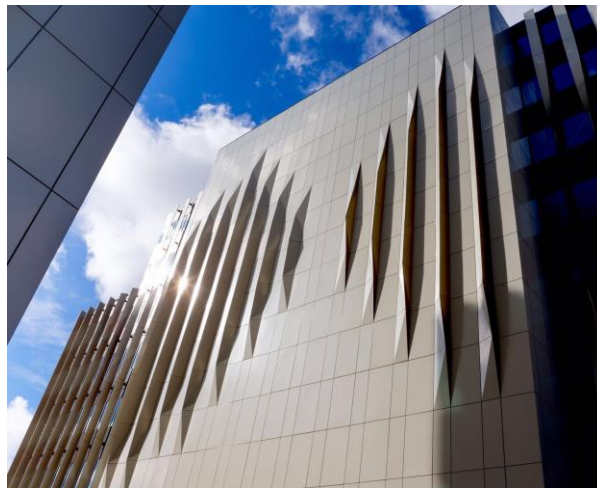
Typical rainscreen façade system
