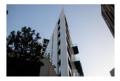
As part of the project, Sotech produced a finite element analysis to prove that the majority of the panels could be manufactured from 2mm alloy whilst keeping deflection within acceptable ranges.
