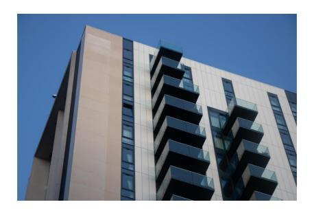
Some 6,500 square meters of Optima FC in an aluminium 1050 Grade with a polyester powder coating finish has been used in the completion of Alto NW06 apartments in Wembley, London.
