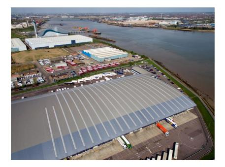
The longest rooflights installed on this huge curved roof are over 118 metres long: among the longest uninterrupted runs ever supplied by Filon Products.
