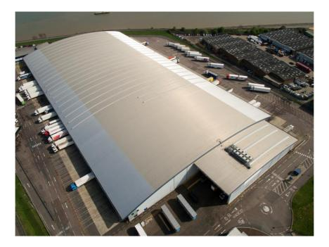
Over 2,600 linear metres of Filon's Monarch F GRP barrel vault rooflights were installed during the refurbishment of this major distribution hub in Belvedere, Kent
