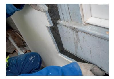
At just 16mm thick, the use of Spacetherm Multi has virtually no negative impact on floor space, making it ideal for refurbishment projects where space is at a premium.
