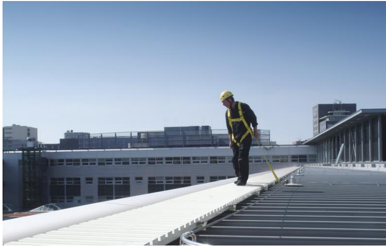
Fig 1: From GD10 Working at heights module: Illustration of cable system and walkway
