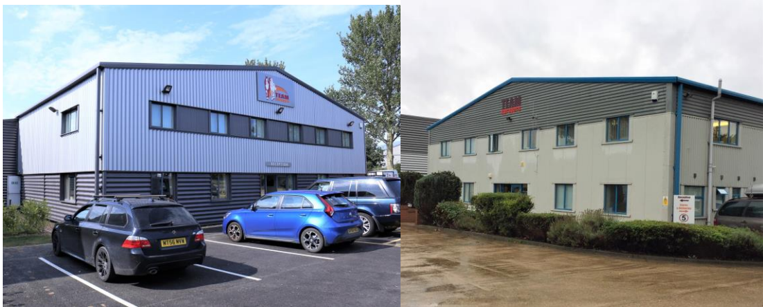
Before and after 'Retrofit Envelope' installation
