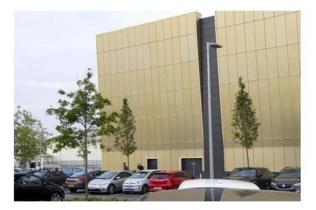
Over 1,200 square metres of Alucobond Silver Metallic 500 and 900 square metres of aluminium anodised Regency Gold 1 have been used in the completion of the White Rose shopping centre in Leeds.
