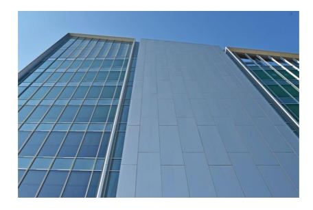
Aluminium Composite Material (ACM) was used for the rainscreen panels due to the size required in order to provide optimum flatness. Due to the size required, panels had to be manufactured in two halves and bolted together as there are restrictions on sheet material sizing.
