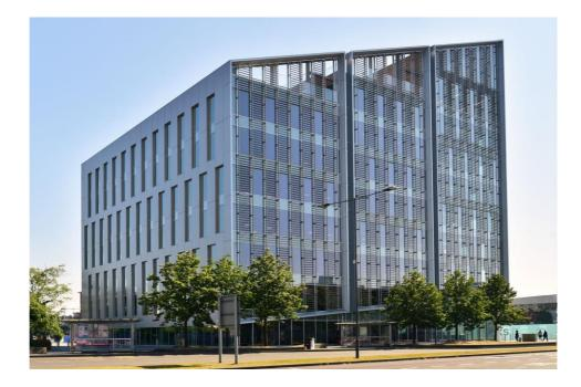
Some 5,500 square metres of a specially designed rainscreen cladding system – a hybrid of Sotech Optima's FC secret fix rainscreen and TFC through fix cassette rainscreen has been used in the  $\pounds$ 450 million regeneration of Slough town centre.
