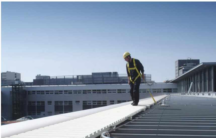
Cable system and walkway
