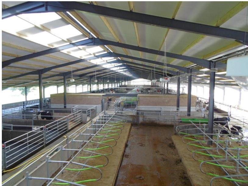
Over 300 square metres of Filon fair assembled insulating rooflights (FAIRs) double skin GRP rooflights have been installed on a new, high technology cow shed with integral milking parlour units at Knott Oak Dairy Farm in Ilminster, Somerset.
