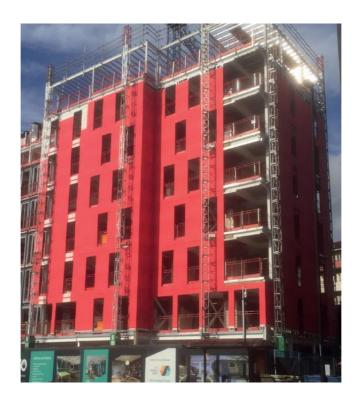
Wraptite® airtightness membrane has been successfully installed on an impressive new luxury high-rise student accommodation project in Newcastle upon Tyne.
