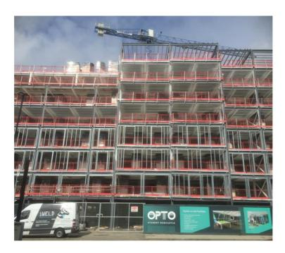
Unlike internal air barriers, which can be complex and costly to install due to the need to accommodate building services such as electrical, lighting, heating and drainage systems, Wraptite was applied externally, quickly and easily to the substrate.
