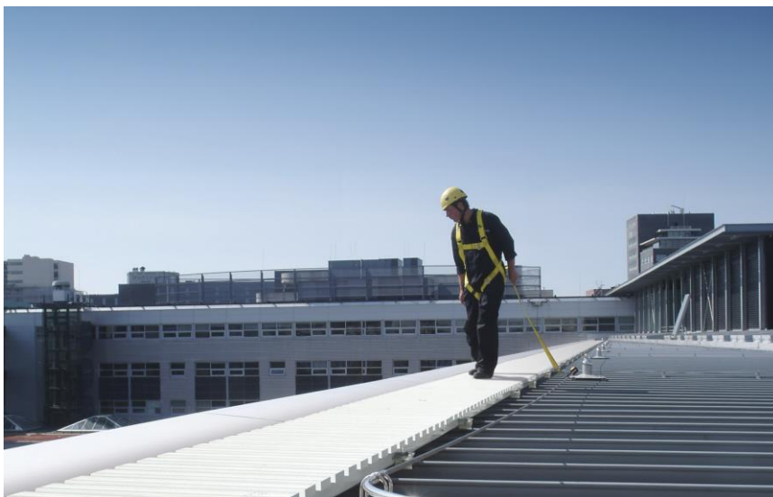
Cable system and walkway
