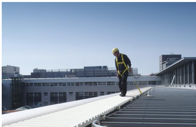
A typical cable system and walkway
