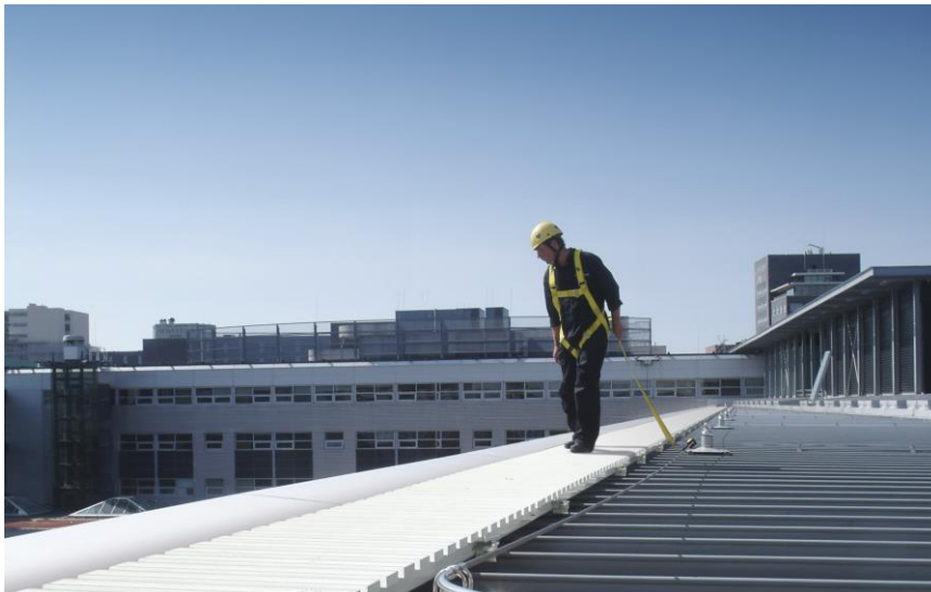
Cable system and walkway
