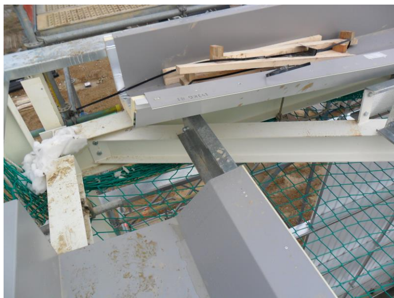
Image 4: Purlin/gutter clash
