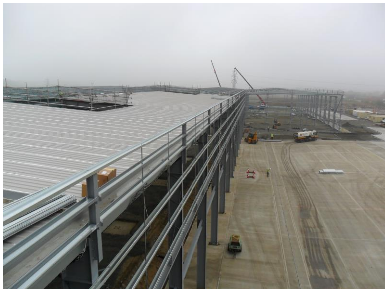
Image 5: Primary and secondary steelwork properly installed
