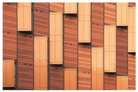
The new appearance of Olympic Way: a rear-ventilated ALUCOBOND® spectra Cupral façade now features an eye-catching metallic shimmer. 1,100 square metres of ALUCOBOND® panels envelop the building.
