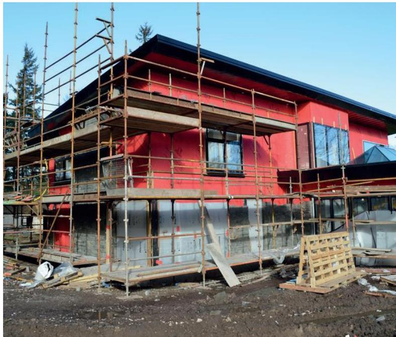
Another key benefit of the system is that the high vapour permeability of Wraptite allows the substrate beneath to dry quickly and moisture vapour to escape. This ensures good indoor air quality and reduces the likelihood of mould, mildew, condensation, timber distortion and metal corrosion.
