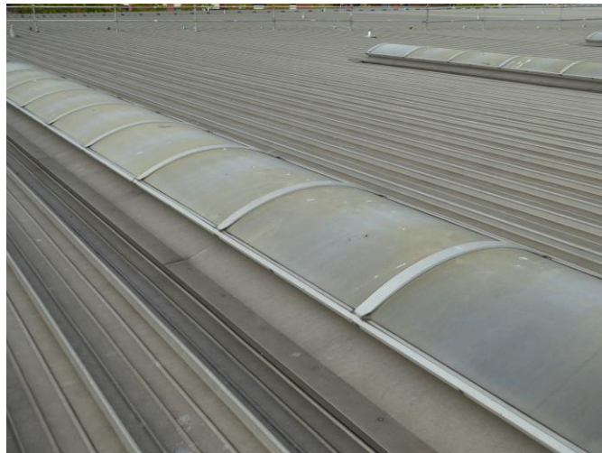
Old polycarbonate rooflights
