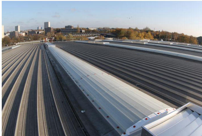
Replaced with Zenon Arc
