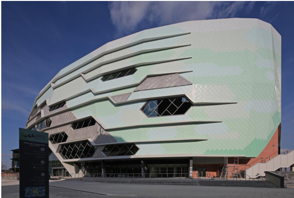
First Direct Arena, Birmingham, Kalzip Limited & SFS Group Fastening Technology
