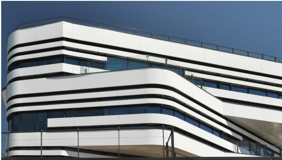
Fusion Building, University of Bournemouth. 3A Composites GmbH Image copyright Paul Scott
