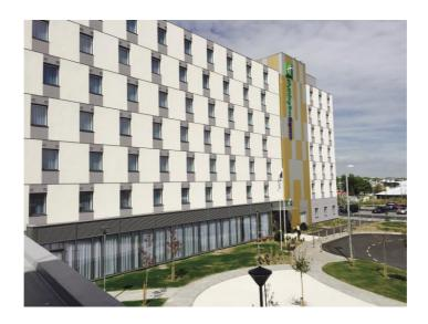
The Crowne Plaza is considered the 'bigger brother'. The concept of a box on a plinth has been developed however, the materials used vary. The front entrance elevation highlights this hotel as a luxury destination whilst projecting ALUCOBOND® cassettes offer a unique prismatic effect to the upper levels.
