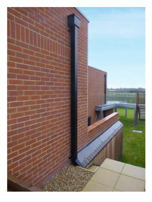
Guttercrest's aluminium rainwater goods have a long life expectancy, in excess of 60 years - enhancing the whole of life embodied energy figure relative to materials with shorter life spans. Aluminium is amongst the most environmentally friendly metals on the planet, with 75% of all aluminium ever produced still being recycled.
