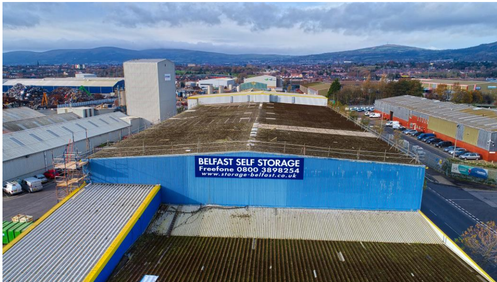
Belfast Self-Storage before refurbishment
