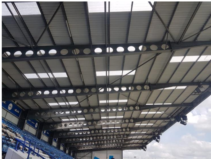
View of rooflights from the stand
