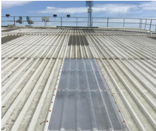
Replacement of rooflight
