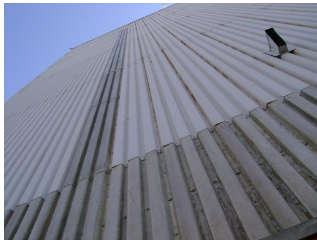
Liebherr Plant before rooflight refurbishment
