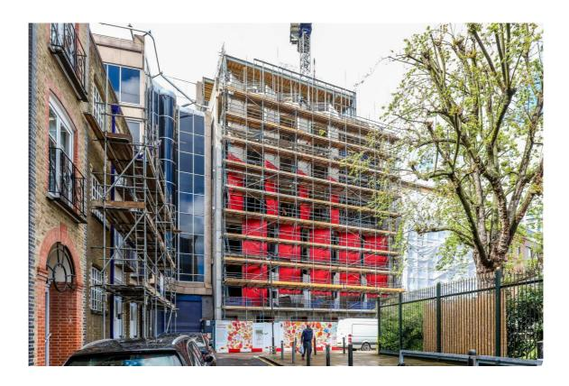
The first external fully adhered vapour permeable air barrier with full BBA certification has been installed as a solution for airtightness, weather protection and breathability at the new administrative headquarters of the Royal College of Pathologists in London.
