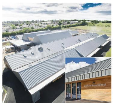
Most of the building is covered with a series of quite steeply pitched Kalzip roofs with valley gutters running between them - slate-clad gable ends blend beautifully with the colour of the cladding sheets.
