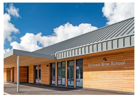
Over 3,000 square metres of Kalzip's new 'Flat Pan' aluminium standing seam profile has been used to clad Orchard Brae School, Aberdeen. Roll-formed onsite, these durable 1.0mm gauge sheets have a 400mm wide rib-less pan - and whilst already used in other locations around the world, this is the first project in the UK where Kalzip's 'Flat Pan' profile sheets have been installed.
