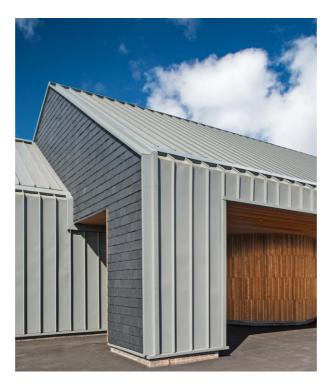
In certain key areas around the building's perimeter, the roof lines have been cleverly extended by continuing the Kalzip 'Flat Pan' cladding sheets down to ground level. This was achieved by first incorporating a composite lined insulated gutter system into the roof just above eaves level before neatly disguising the gutters behind a bespoke fascia flashing.
