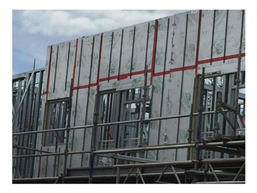
The impressive performance of A. Proctor Group's Wraptite Tape, which provides a vapour permeable air barrier has been successfully used on a new care home in the historic city of Edinburgh.
