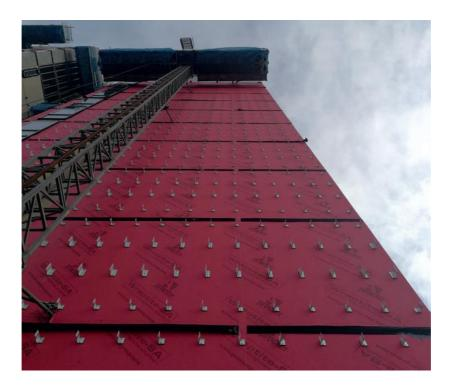
Stephen Hull, Director of InOpera Facades, commented: "Modelling the intended construction with the use of Wraptite, highlighted the ability to improve airtightness whilst reducing the depth of rainscreen support system and insulation. The use of a standard membrane would have required a greater emphasis on this, therefore increasing the overall component cost of the project. Minor cladding zone increases on a project of this height can have a huge effect.
