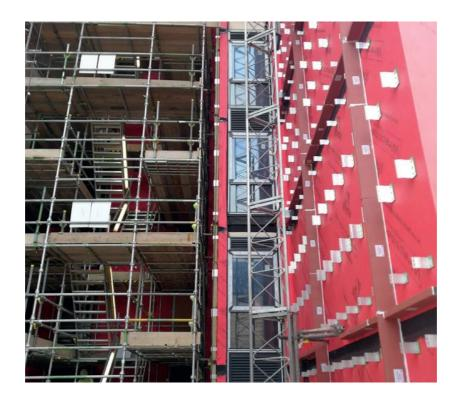
The Wraptite self-adhesive membrane was applied externally, quickly and easily ensuring a higher quality installation, and a more robust through wall rainscreen cladding system."
