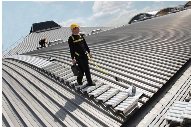
*Latchways Constant Force fall protection and WalkSafe system on Kalzip standing seam roof. Image courtesy of Latchways plc*
